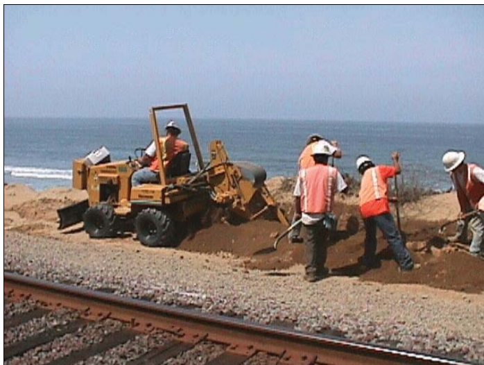
The construction crew digs trenches for sensed cables.
